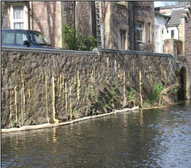
Picture 3: Resin emerging through the flood wall.
