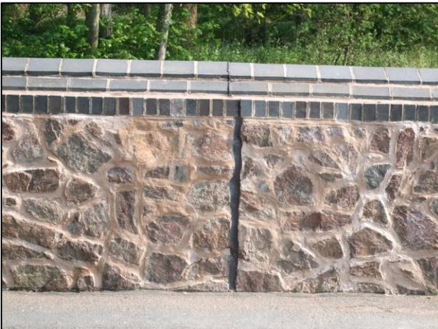
Picture 4: Finishing work included re-cutting expansion joints and re-pointed stonework.
