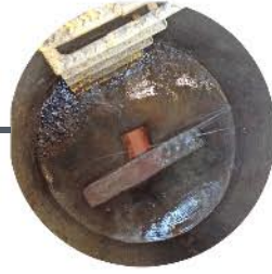
Leaking manholes
