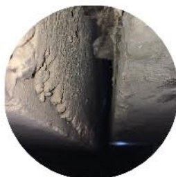
Expansion joint repairs & leak sealing
