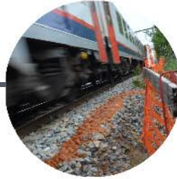
Stabilisation of rail ballast
