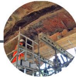
Bearing repairs
