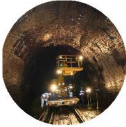
Leak sealing to bridges, tunnels & underpasses
