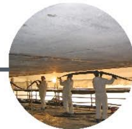
Carbon fibre installation
