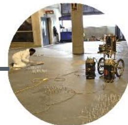
Epoxy void & crack injection
