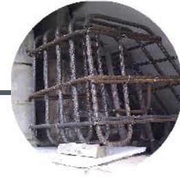
Bridge bearing replacement
